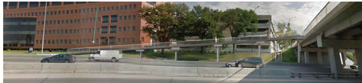
Elevated Pedestrian Accessible Structure - north of Portage Avenue
