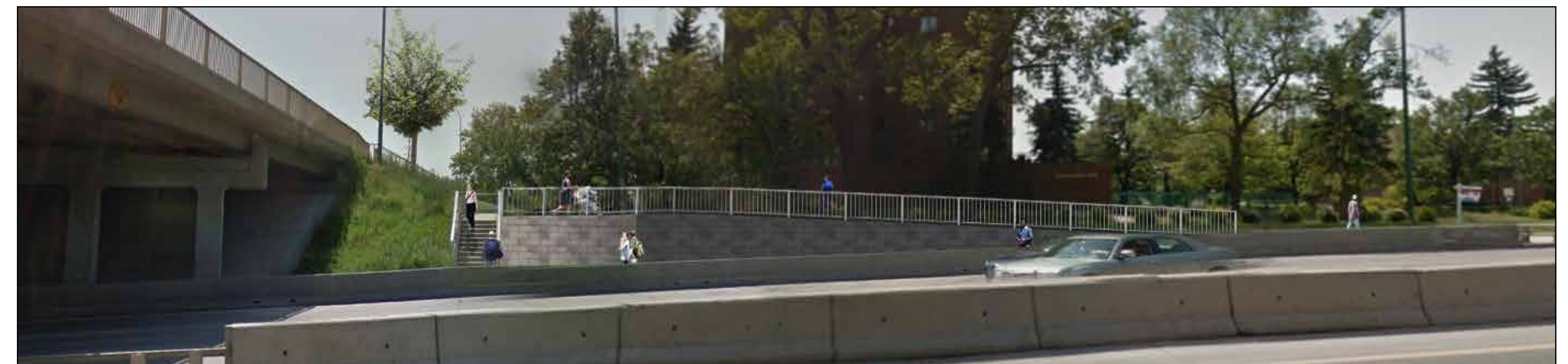
Accessible Pedestrian Route - south of Portage Avenue
