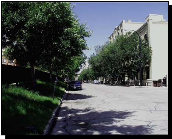
Streetscape 5. Bannatyne Avenue looking west from Ship Street toward Main, with Donald Bain and Merrick Anderson buildings on right.
