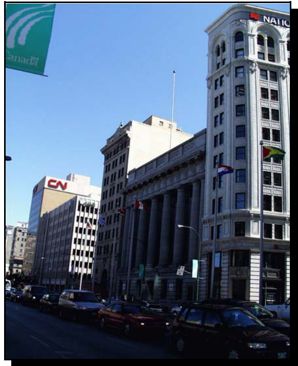
Figure 5 b. Former temple-like Bank of Commerce building set between two early skyscrapers on Main Street (Parks Canada, July 1999).
