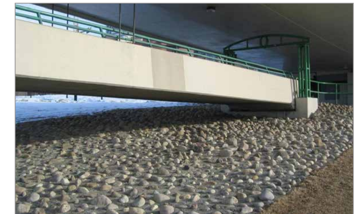
Textured surfaces to discourage loitering under the bridge
