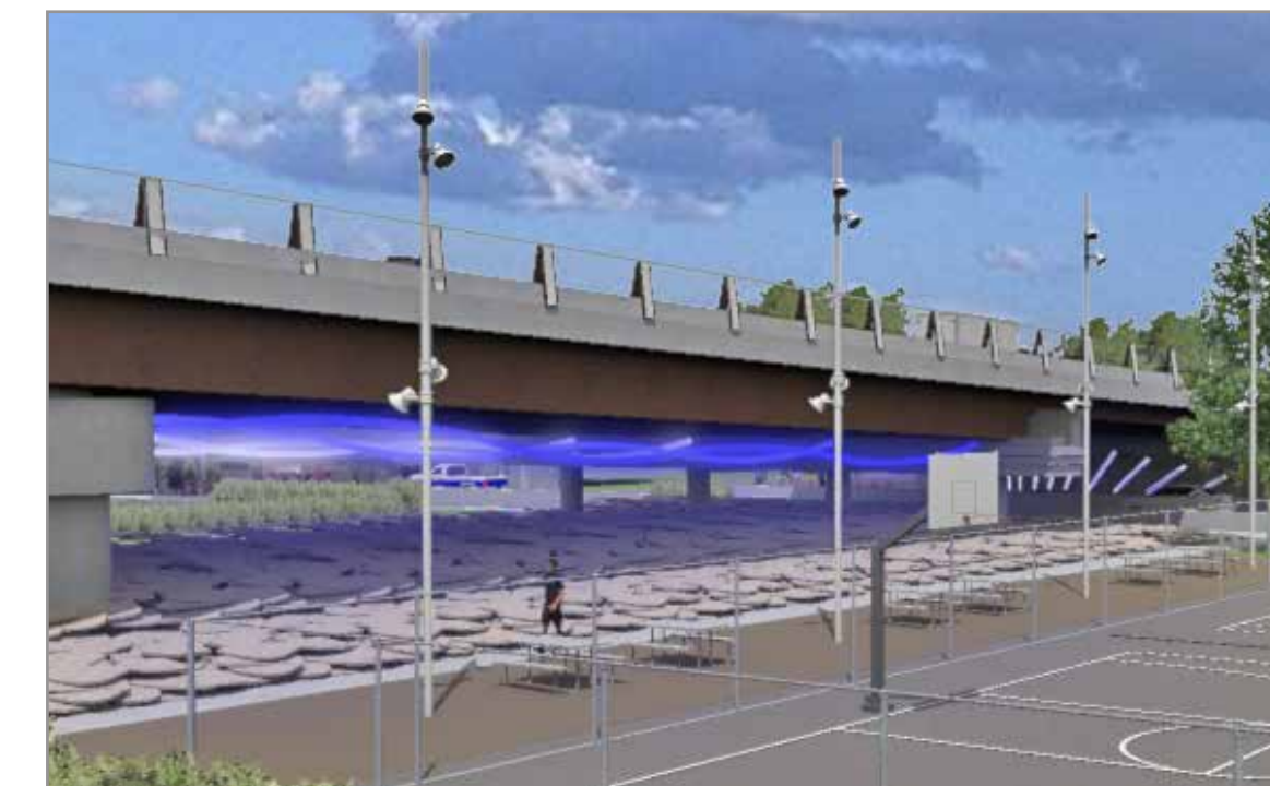
Decorative and safety lighting and SafeWalk call stations on, under and around the bridge
