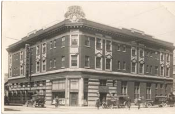
St. Charles Hotel, ca.1913 shortly after opening. Note the alternating stone and brick bands on the ground floor.
