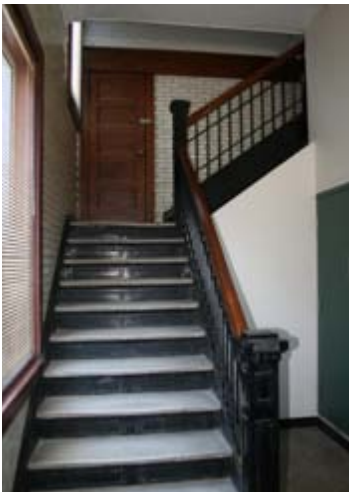
Main staircase (northwest corner) to second floor.
