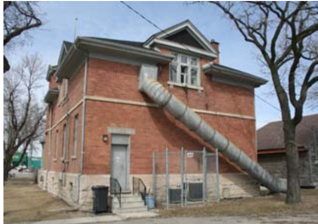
Rear (south) façade with the metal fire escape tube.
