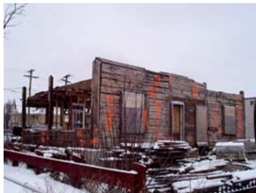
Dismantling of Royal House, November 2000
