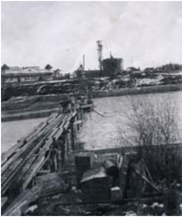
This 1918 photograph from the Winnipeg side of the Red River shows the St. Boniface Surge Tank under construction.
