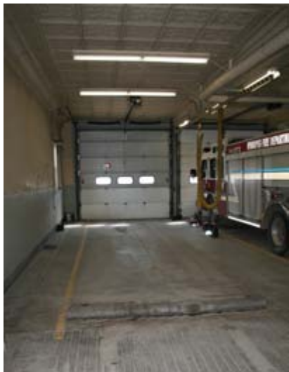
Apparatus bay with original tin ceiling and ribbed concrete floor.
