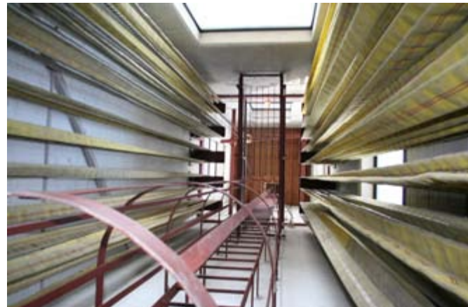
Looking up into the hose drying tower.
