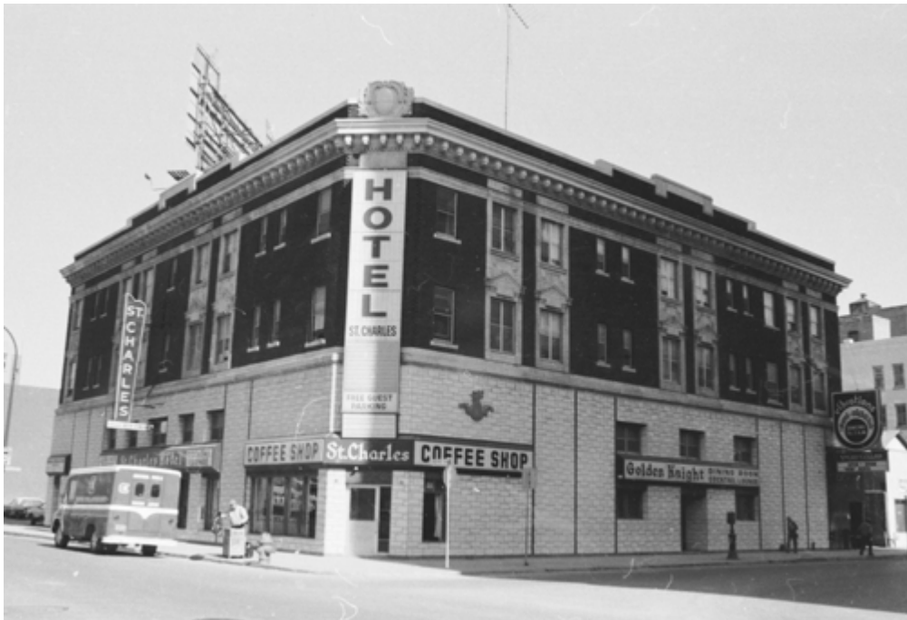
St. Charles Hotel, ca.1974 with the tile cladding attached to the ground floor walls.
