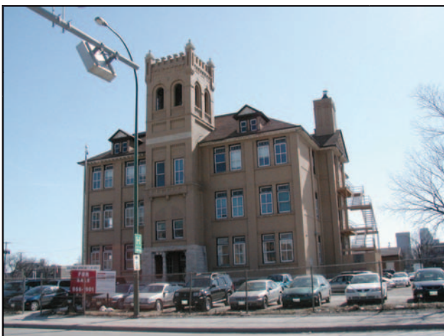
Former Sacre-Coeur School No. 2 (I.B. Somerset School), 775 Sherbrook Street, vacant
