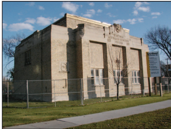
Women's Tribute Memorial Lodge undergoing stabilization
