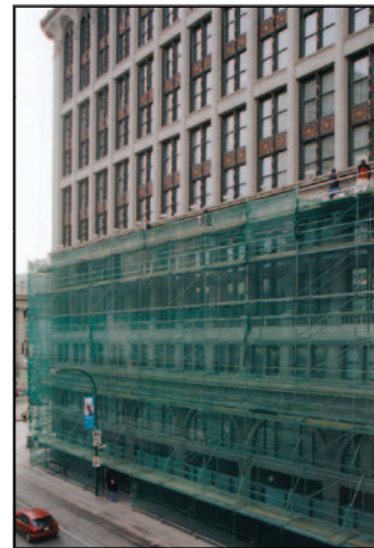
Scaffolding used for terra cotta repair, Paris Building
