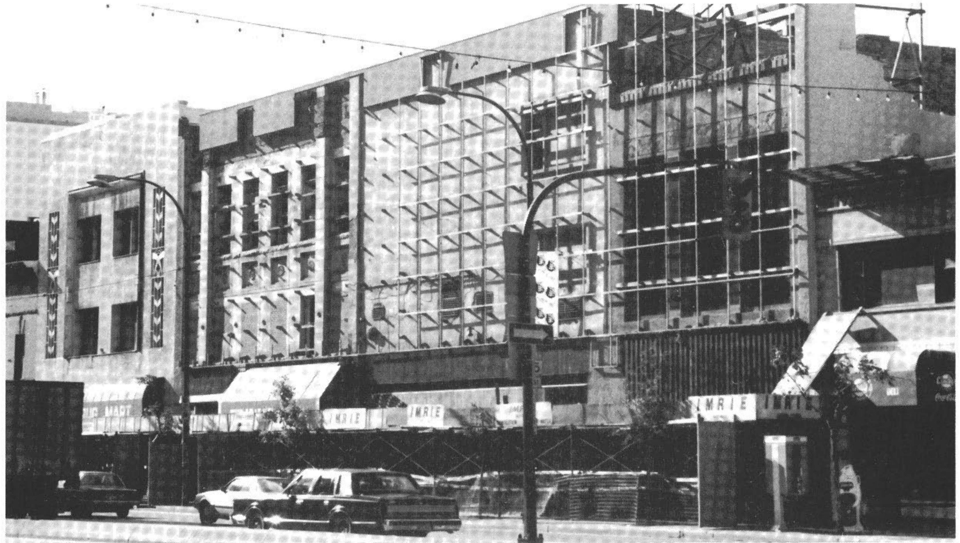
The demolition of 287 - 295 Portage Avenue, 1991. City of Winnipeg
