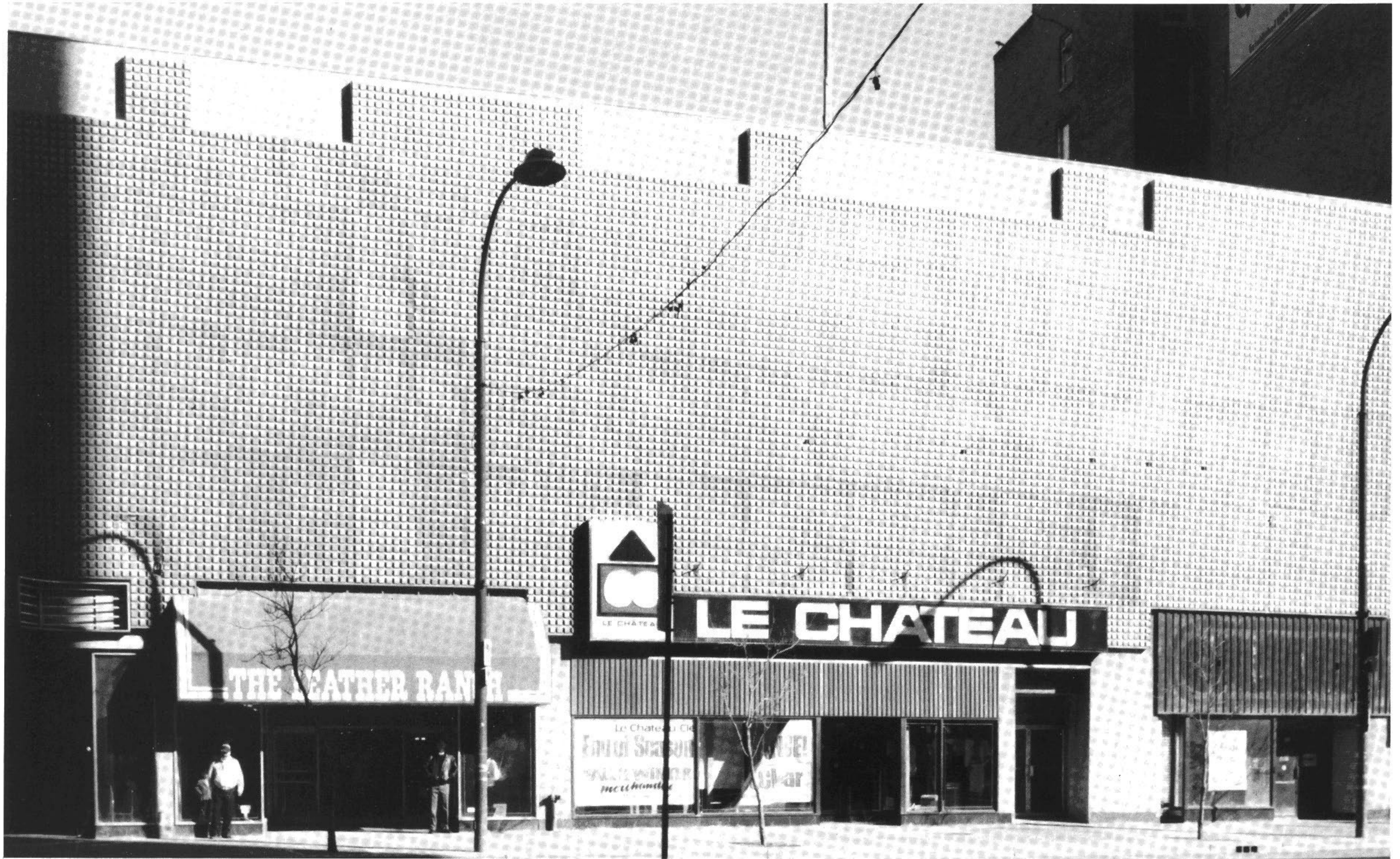
The Genser Building prior to demolition, 1991. City of Winnipeg
