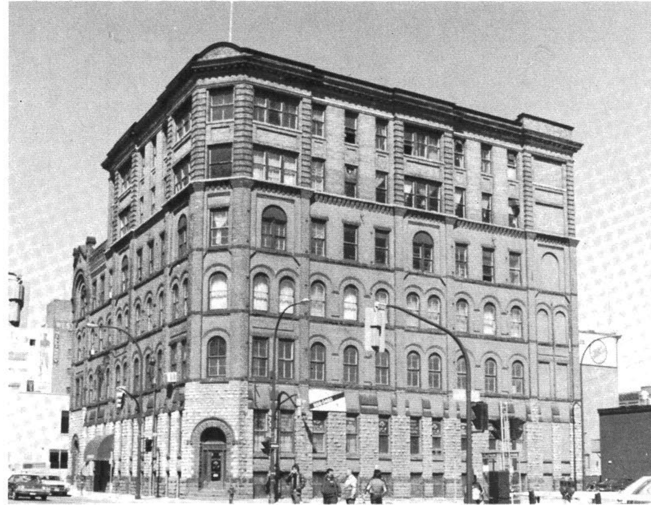
The Peck Building in 1984.
