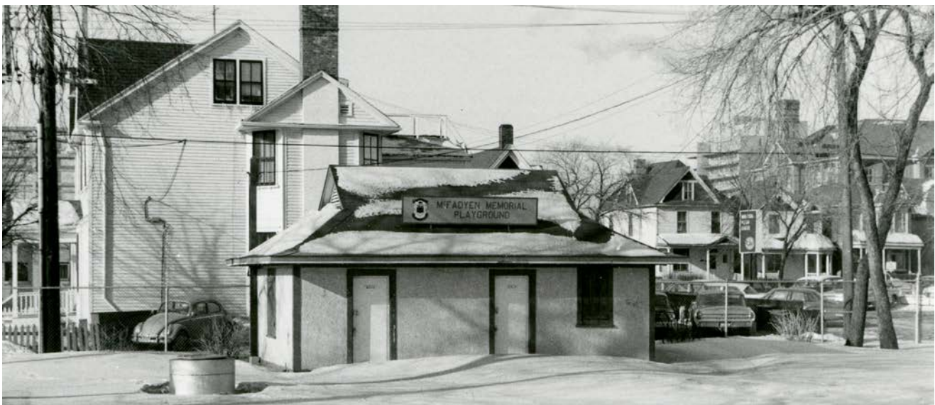
McFadyen Memorial Playground, formerly located on the northwest corner of Hargrave Street and York Avenue, 1968. It was relocated to Assiniboine Avenue in 1972.
