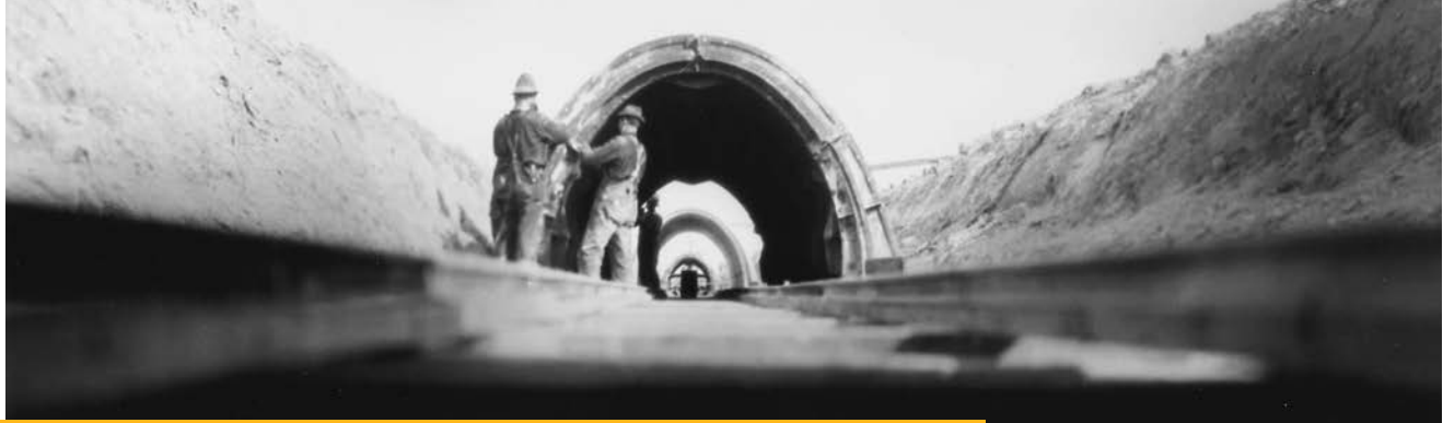
Three sections of arch as viewed from invert, August 31, 1915. (Aqueduct)
